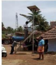
Rural Energy Systems
